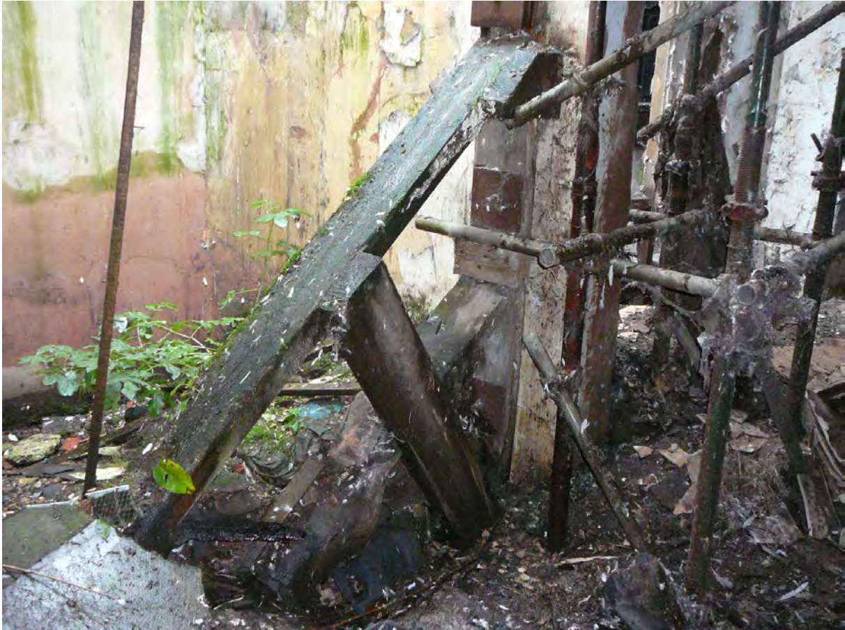
Photograph 6: Raking shore to support for steel beam
