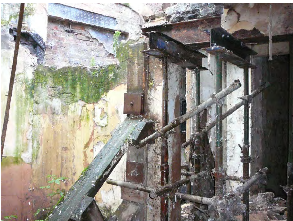
Photograph 4: Propping to steel beam
