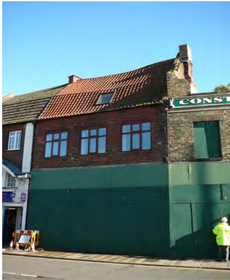
Photograph 1: Intact portion of Nene Quay
