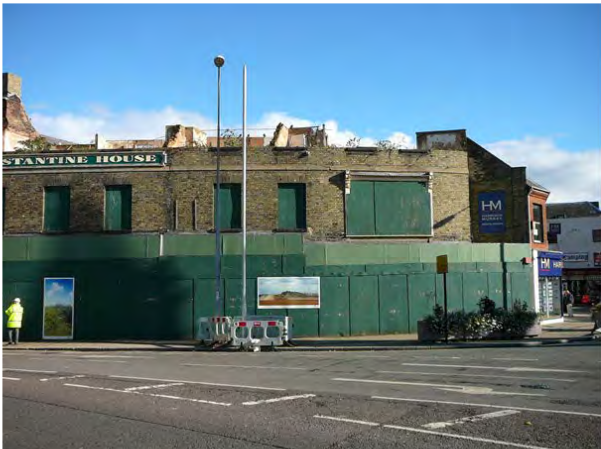
Photograph 2: Part demolished portion of 1 Nene Quay
