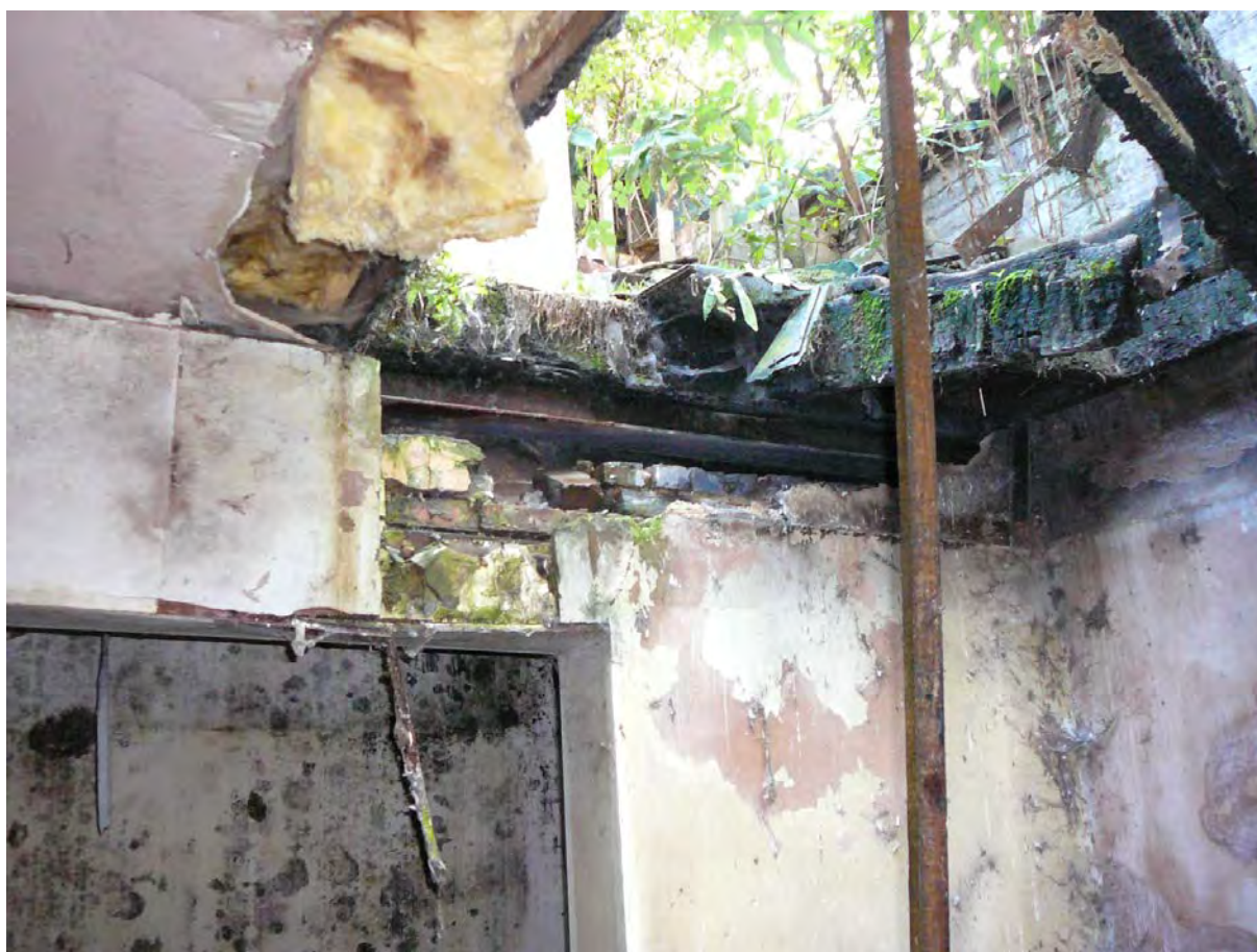
Photograph 3: View through first floor
